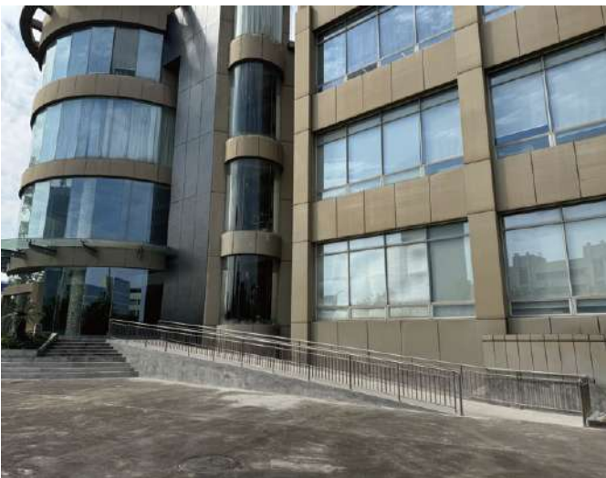
Barrier-free access ramp
