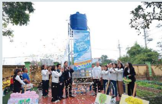
Building clen water tank with Carter’s & Planet Water
